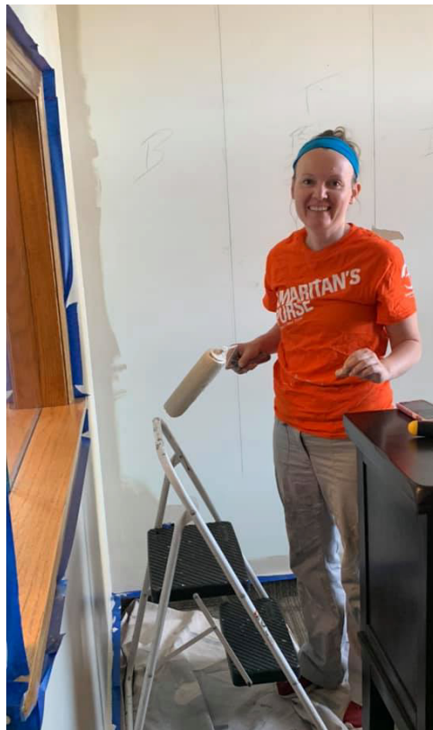
Many volunteers helped repaint interior rooms.
